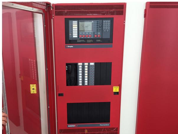
**FIRE PANEL:** This houses alarm controls for the overall facility. This device allows for pinpointing alarm locations and provides direct communication with the fire department.
